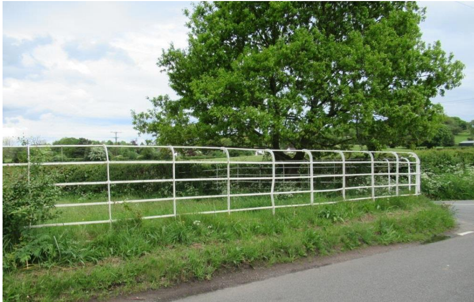
Figure 6.26 Cheshire railings in Chorlton parish
