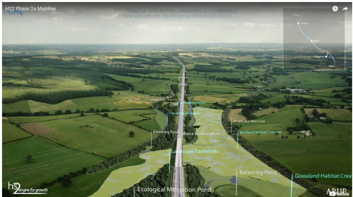
Figure 7.4f Approach to Whitmore Heath tunnel south portal: Meece Brook viaduct and embankment in Meece valley; Bent Lane on the left, WCML and isolated settlements of Hill Chorlton cluster hamlet on the right.
