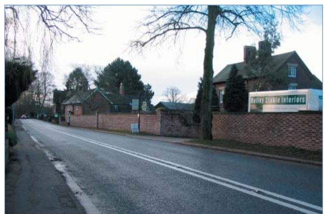
Boundary wall to Betley Court Farm
