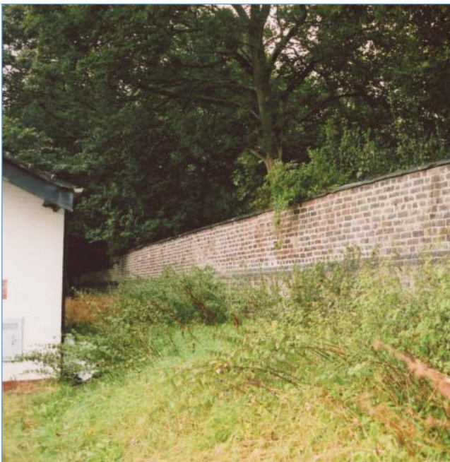
Former wall to Betley New Hall
