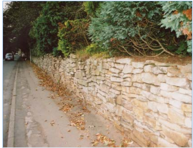
Sandstone walls in Main Road
