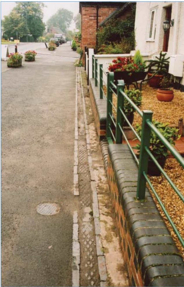
Staffordshire blue brick paviors next to the Reading Room
