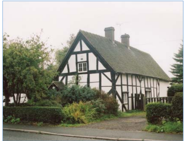
Timber framed cottage in Main Road (Rose Cottage)
