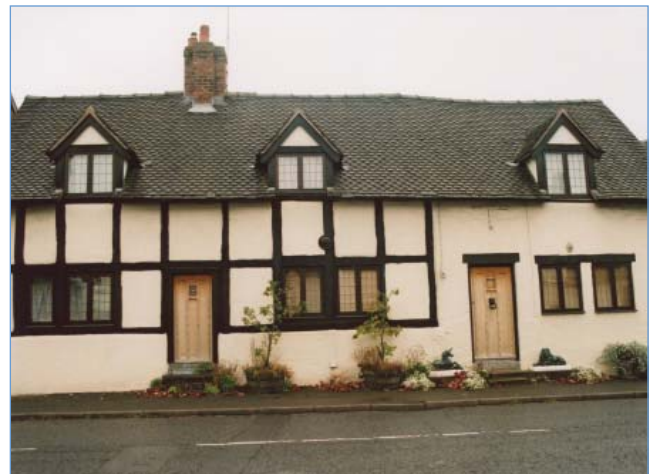
Examples of the use of scalloped clay tiles in Main Road (Hawthorn Cottage and Tudor House)
