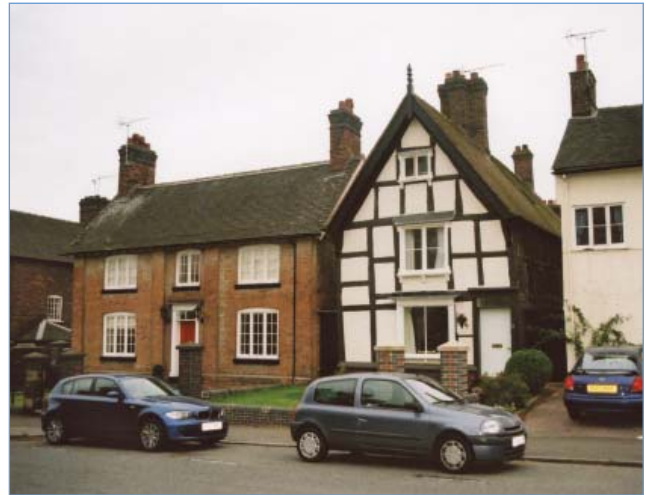
This listed timber framed cottage lies at right angles to Main Road
