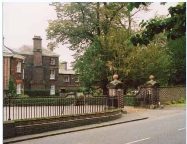
Betley Court boundary walls and railings
