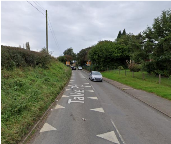
Figure 2: Picture of current speed arrangement along Talke Road
