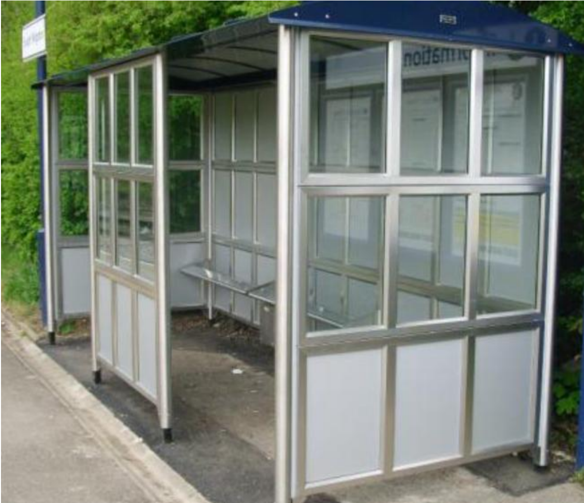
New waiting shelters on platforms 1 and 4
