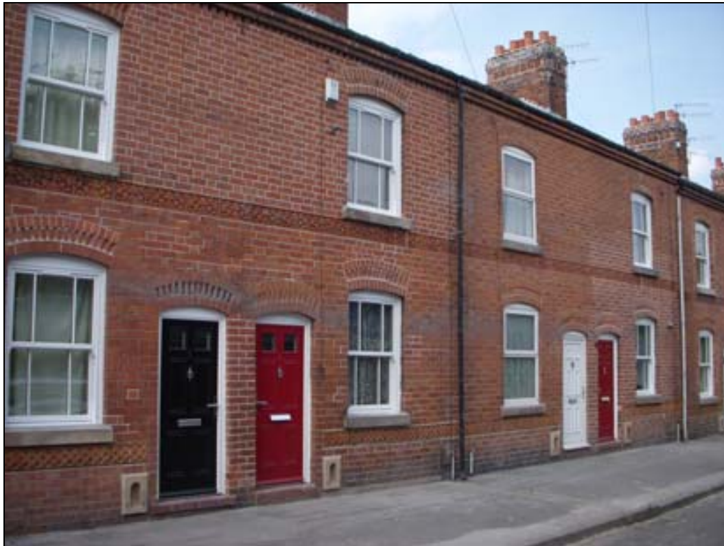
Figure 9: Knutton Heritage Scheme facelift works:
