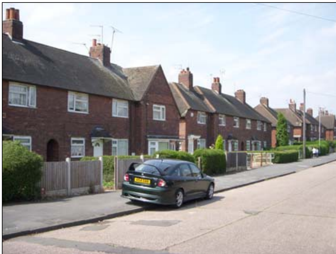
Figure 6: Typical 1940's/ 1950's Housing common throughout Cross Heath:
