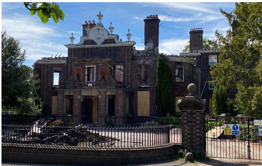
Betley Court after the fire
